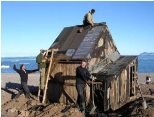
Elvsborg: Start and half way. From the lower edge of the window and up, the major part is original.
