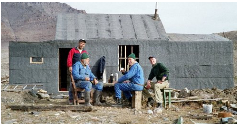
The outer felt has been put on the walls, but the roof isn't quite finished. The inner felt has been nailed on vertically, and the outer felt welded on horizontally. From left: Knut, Ivar, Otto and Anders
