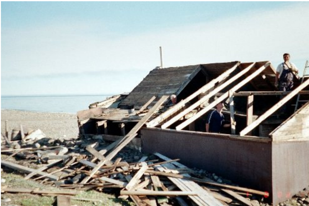
Taking down the provisional porch. It contained a number of reusable materials
