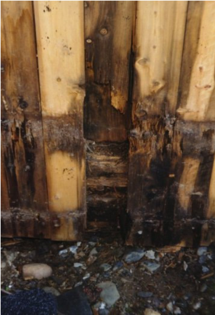
Photo: Here the rottenness must be removed and new boards put in.
