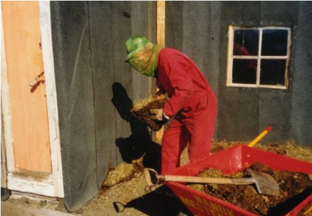
Thor builds a new dirt wall
