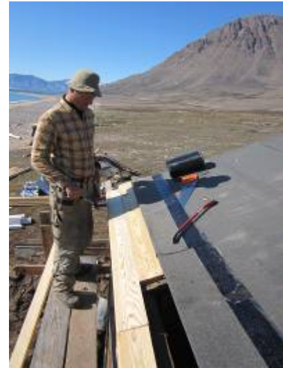
Left: Cleaning the kitchen area. Right: Repairing the roof base and roofing with felt.
