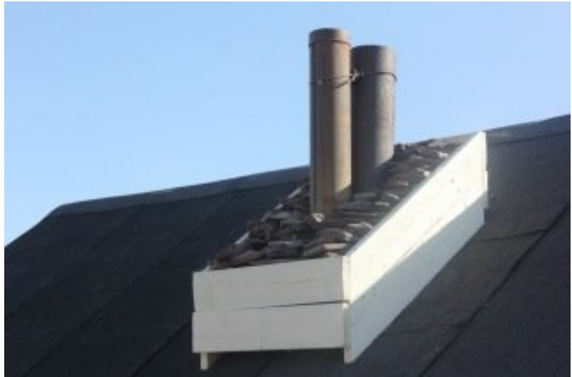
The chimney before and after renovation.
