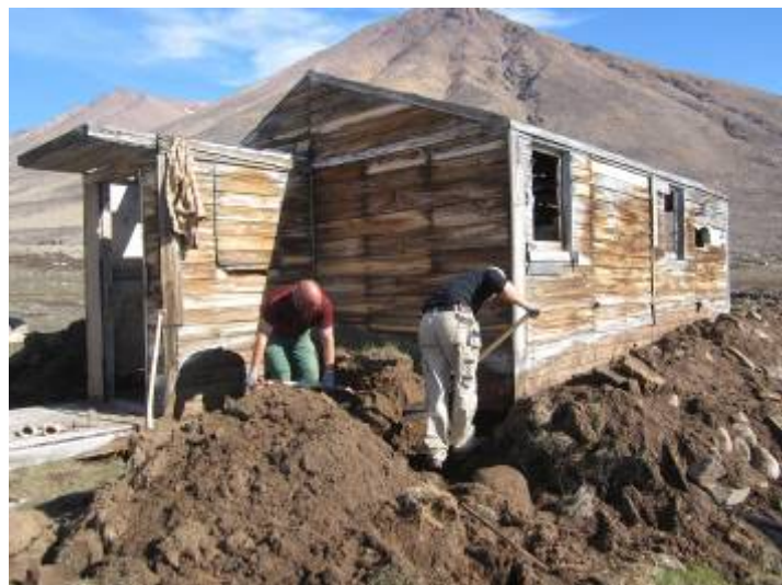
Left: Soaked træfiberplader. Right: The house is dug free to dry.
