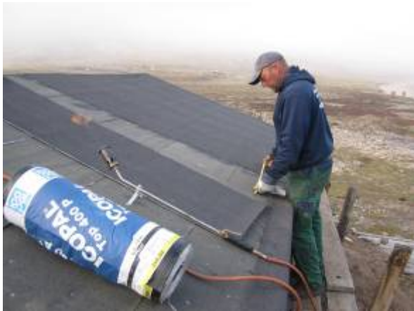
Left: The roof is given new roofing felt. Right: Completed gable.
