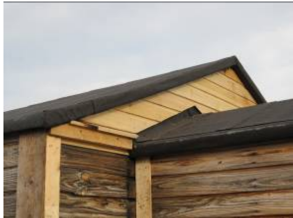
Left: The roof is given new roofing felt. Right: Completed gable.
